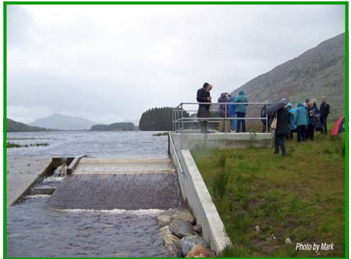
Loch Gynack, the source of the river. The weir providing hydraulic head for the Pitmain generating station is in the foreground
