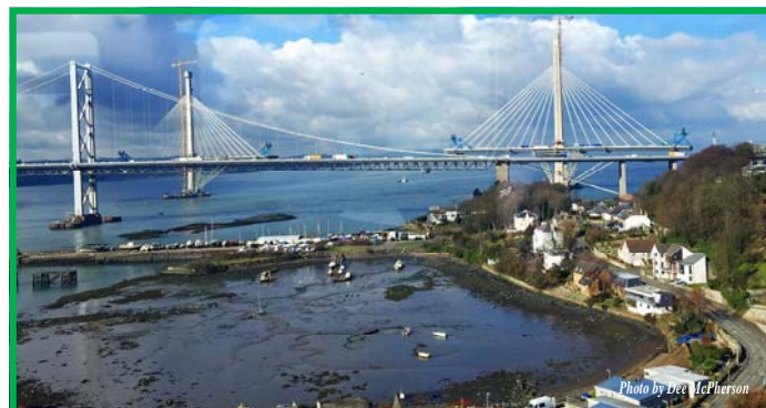
Road bridges across the Firth of Forth. The suspension bridge closest is the original one. The more distant cable stay bridge is the new Queensferry Bridge under construction
