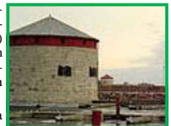
One of three Martello Tower redoubts. A post -1812 fortification found at Kingston
