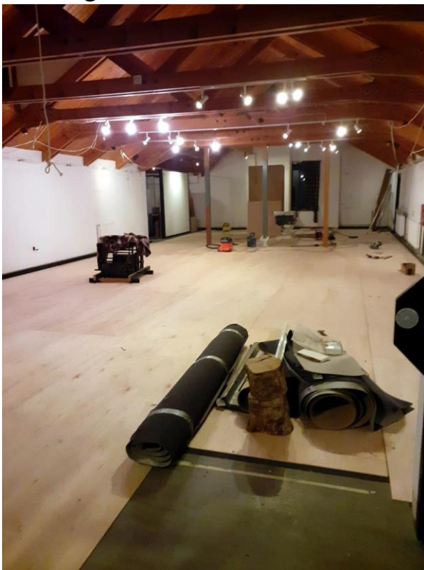
Refurbishment looking south
