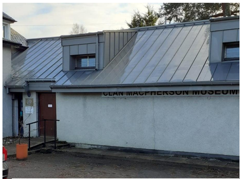
New roof from car park
