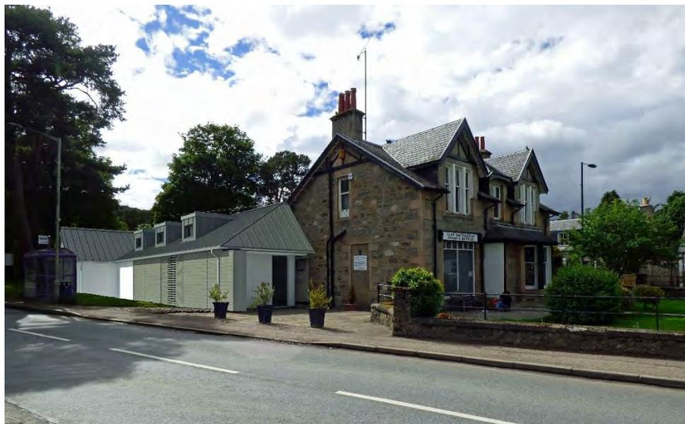
Option 1. Replace the existing roof cladding of tiles with much lighter zinc and include insulation. The roof overhang to be extended considerably in order to clad the walls in the future and allow for excess rain water from the roof to avoid the walls.
